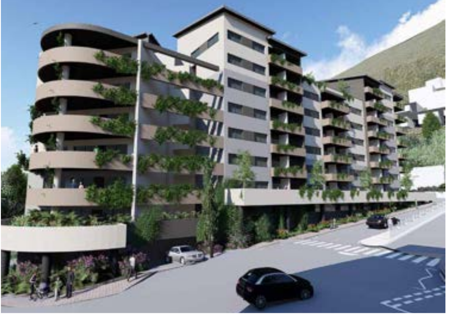
The Queen's Views Development, a mixed use scheme with rental, affordable and cultural facilities
